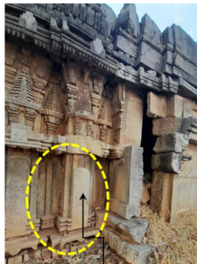
Outer wall composed of vertically placed single stone slabs intended for carving.
